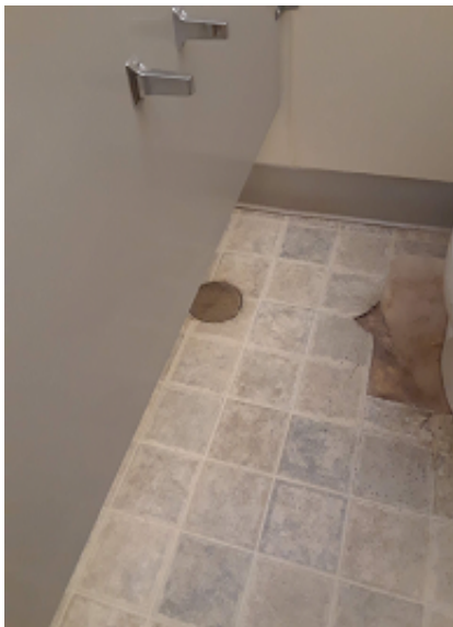
Wing 1-4: Staff Restroom (HM#21)
